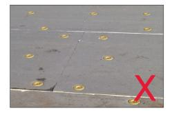
Snap chalk lines to lay-out fastener grid pattern for field, perimeters, and corners.
